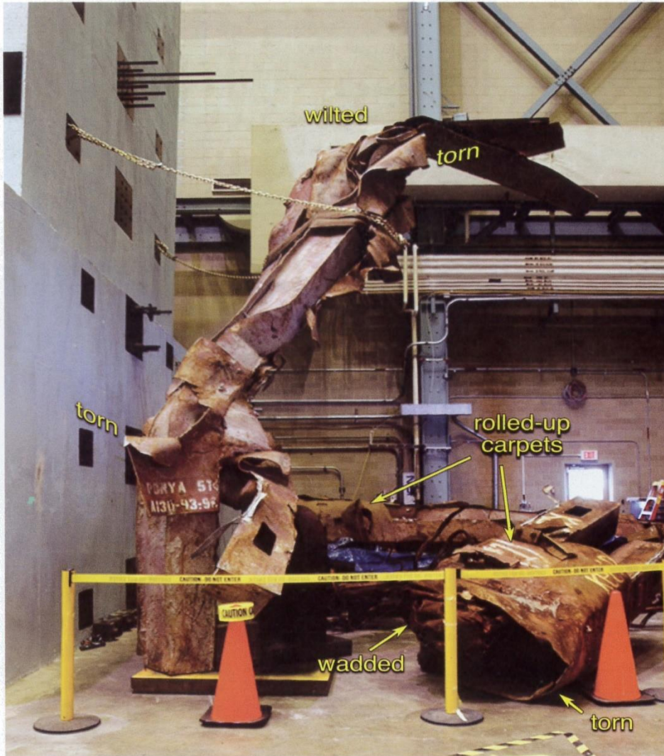
Figure 372. Steel columns from the WTC that look like paper maché. 169
