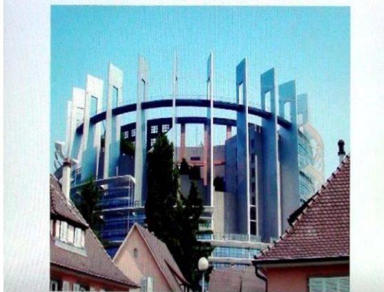
Louis Weiss Building, The European Parliament, Strasbourg France – designed to resemble an unfinished tower
